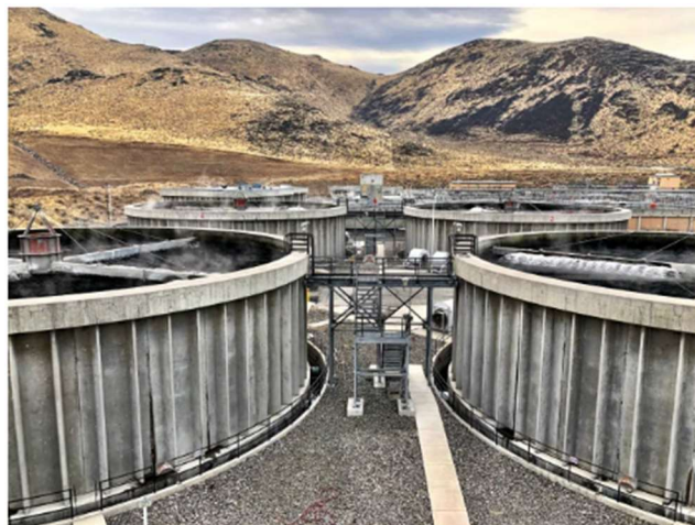
Figure 13 TMWRF facility, via TMWRF website
